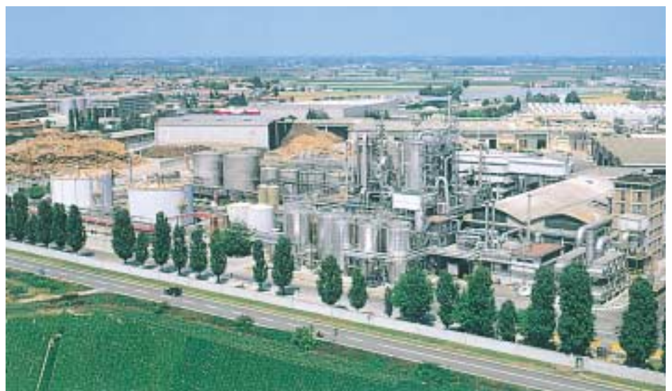
One of Sadepan's plants – note the wood depot (far left): it's all recycled!
